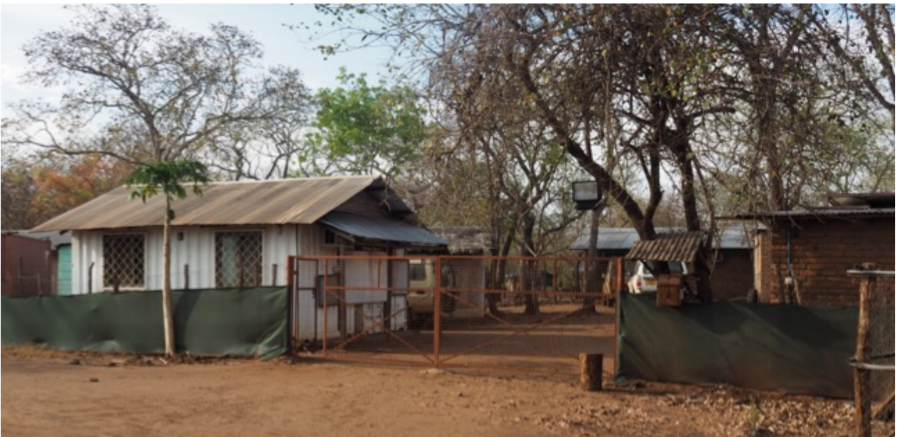
Figure 5 – Ntaka Hill camp offices
