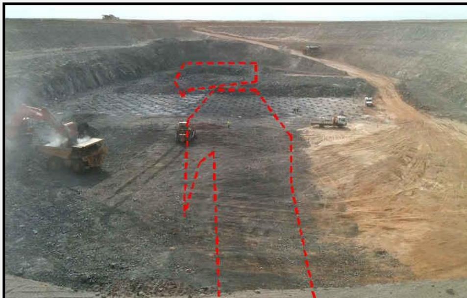
Figure 2: Starter Pit at end of September, looking east showing projected ore boundary on 120RL
