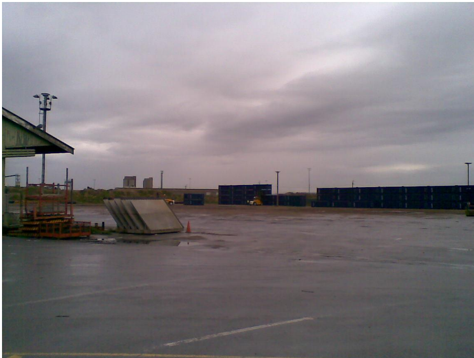
Photo 3: Containers in Storage Area
