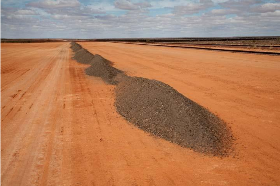
Photo 3: Initial Stockpile Establishment Rankin Dam
