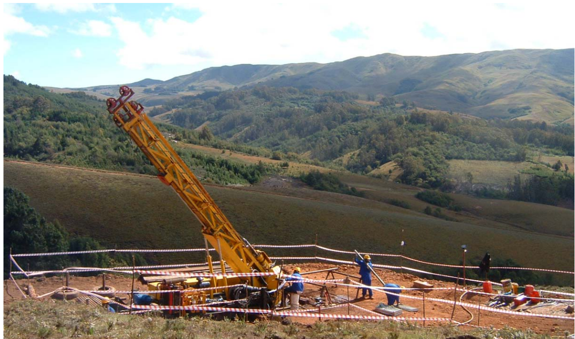
Drilling NDH020, Nkenja East Area, Luwumbu
